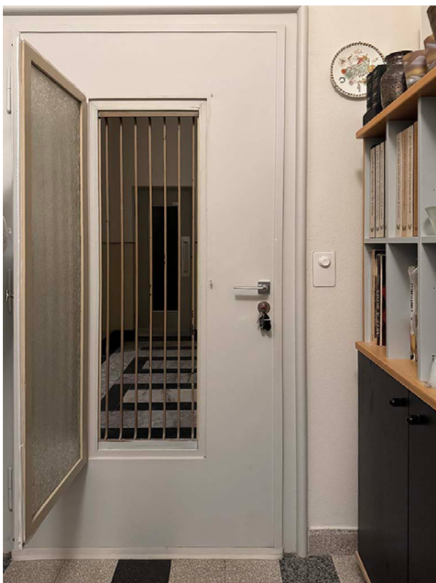
Entrance door from the inside, with the window open.
